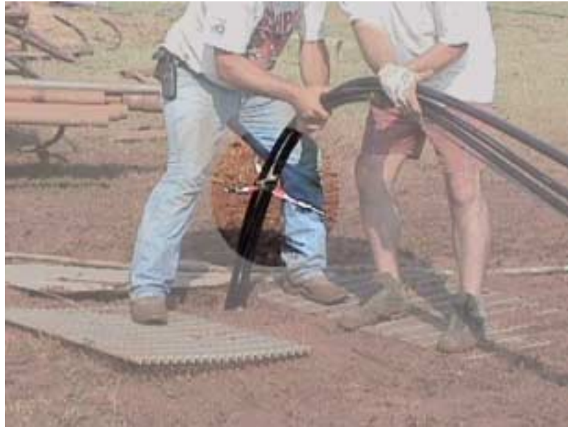
Figure 1a. Thermistor system during installation.
